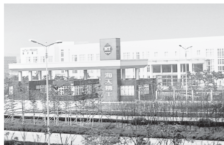
Ningbo Dagang Production Base
