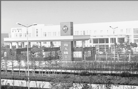
Ningbo Dagang Production Base
